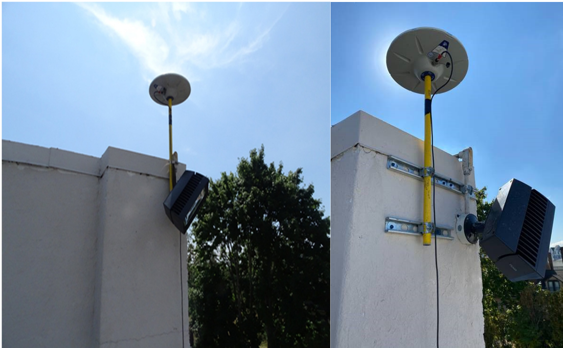
Figure 4. OSNR’s original antenna position (left) from 07/25/2020 (DN207) to 10/02/2020 (DN276), and OSNR’s antenna position following the position shift that occurred on DN 276 (right). The antenna remained in the shifted position through the end of the project.
