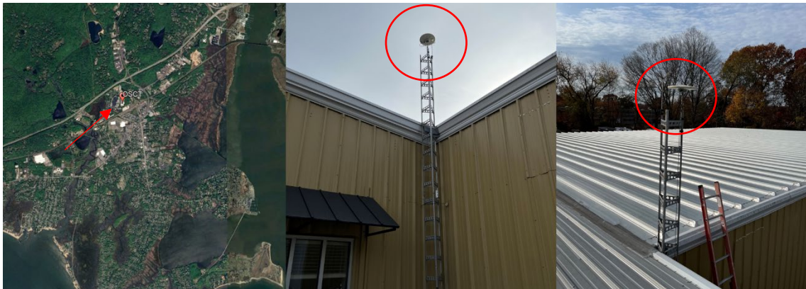
Figure 2. Ortho imagery and setup images of OSI’s user-installed base station “OSCT” on the roof of Ocean Survey’s home office in Old Saybrook, CT.
