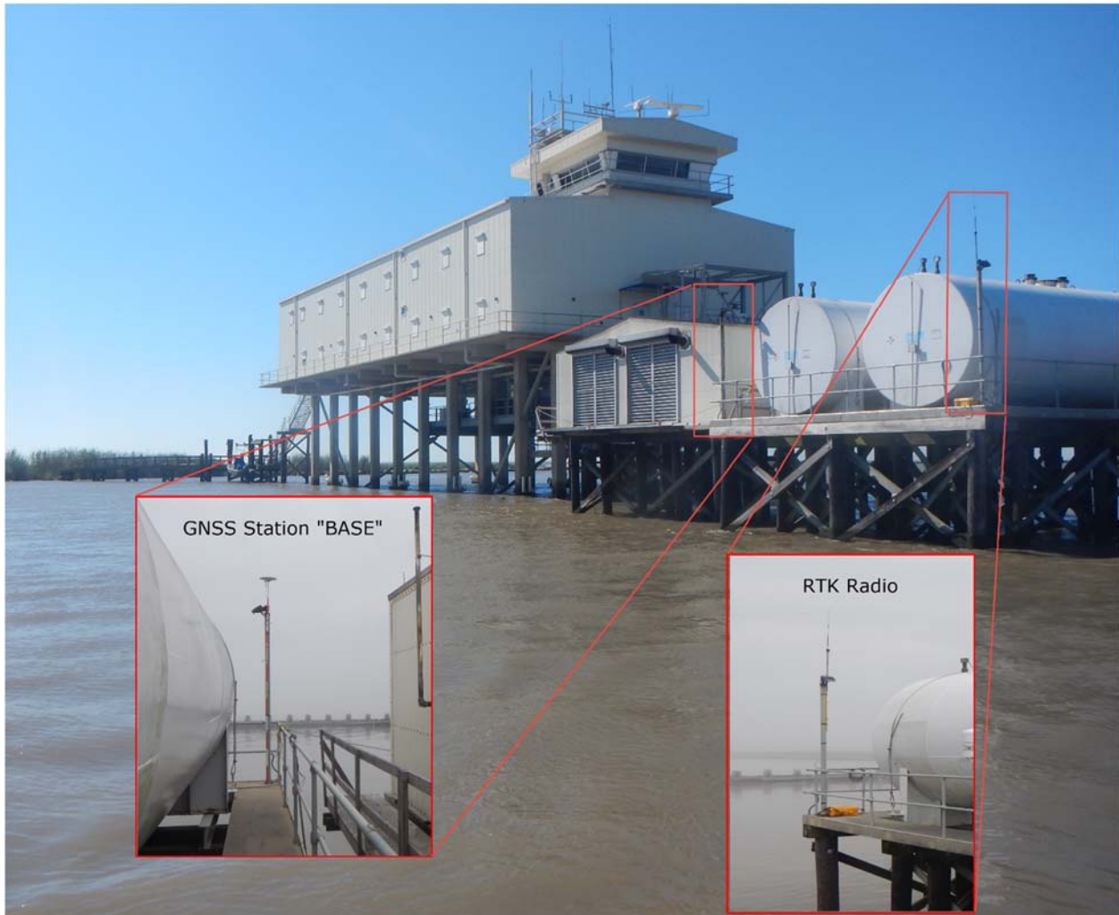
Figure 5. DEA Installed GNSS Station "BASE"
