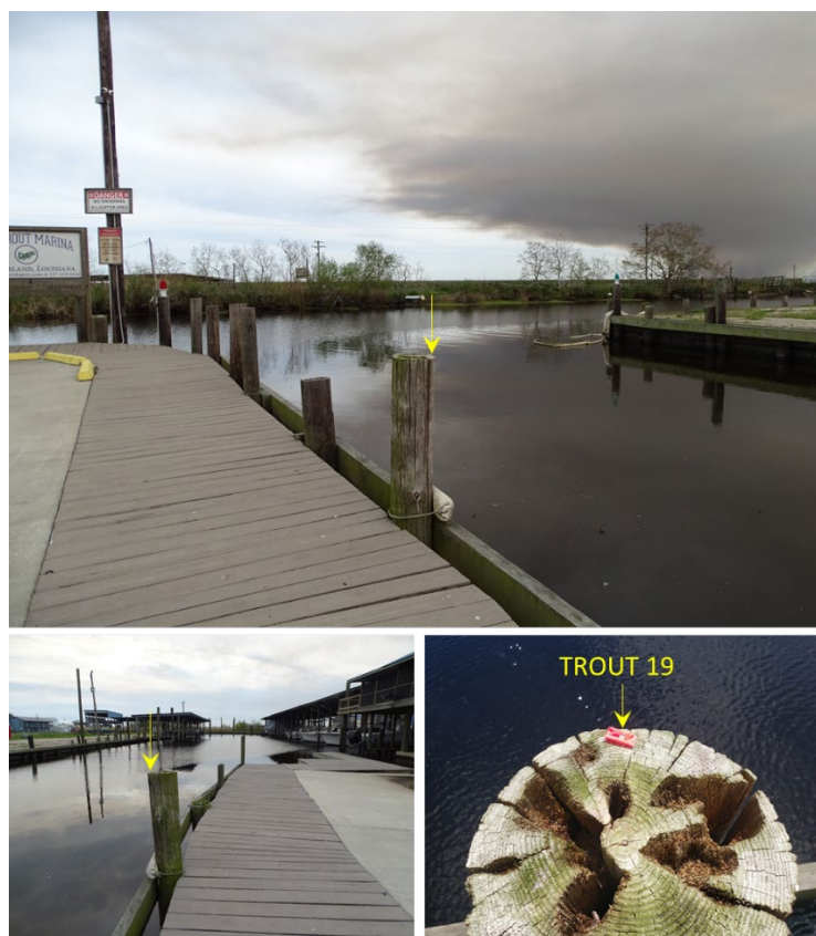
Figure 7. TROUT 19 is a pink flagged PK Nail in a dock piling at Sea Trout Marina in Pecan Island. This point was used exclusively by the R/V H.F. Stout .
