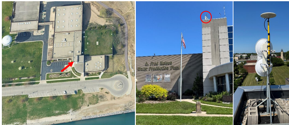
Figure 2. Ortho imagery and setup images of OSI’s user-installed base station “OSKE” on the roof of the Kenosha Water Production Plant in Kenosha, WI.
